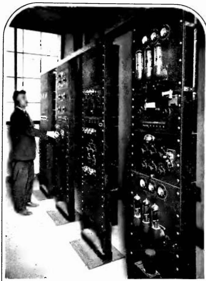
THE LOW-POWER UNITS
