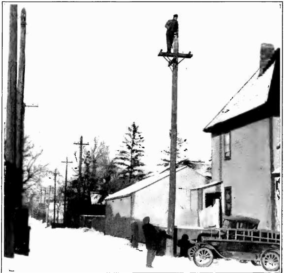
INSTALLING AN ANTENNA IN WINNIPEG, MANITOBA The local telephone company grants the right to use a telephone pole for $6 a year and their linemen erect the antenna for a small sum
